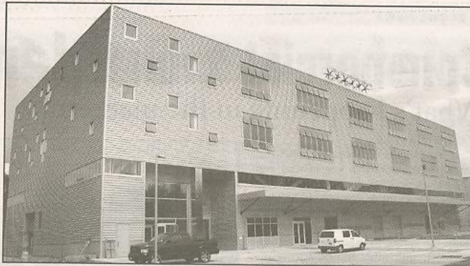
The Perry Building at the Brooklyn Navy Yard will be awarded the inaugural National Grid Award for Energy Conservation.
